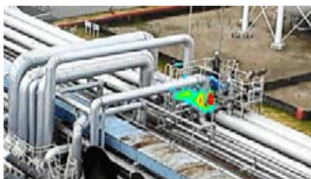
Gas leakage detection using high-performance camera
